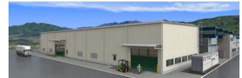
Ayabe Fastener Plant Restructured factory
