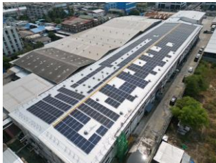
Solar panels (Subsidiary in Thailand)
