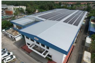
Solar panels (Subsidiary in Malaysia)
